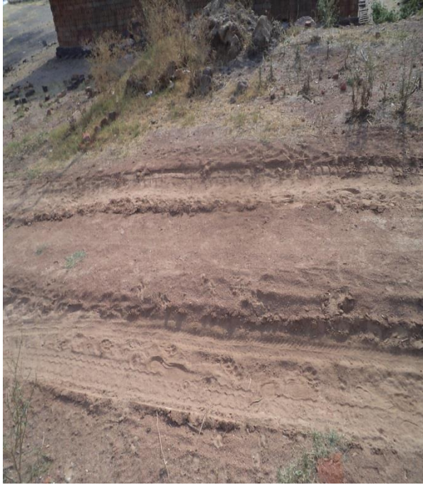
Fig.7: Showing the damaged roads due to transportation Coal and manufactured bricks
